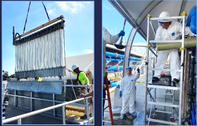
Replacement of membranes
