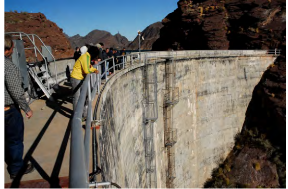
Metropolitan’s dams are inspected on a regular basis.
