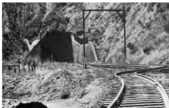
Examples of surface fault displacement. The photograph on the left shows railroad tracks displaced as a result of the 1952 M7.5 Kern County Earthquake. The photograph on the right shows a field that shifted as a result of the 2010 M7.1 earthquake in Canterbury, New Zealand.
