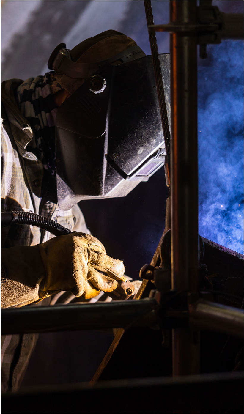
Welder at work during a pumping plant shutdown in the Desert.
