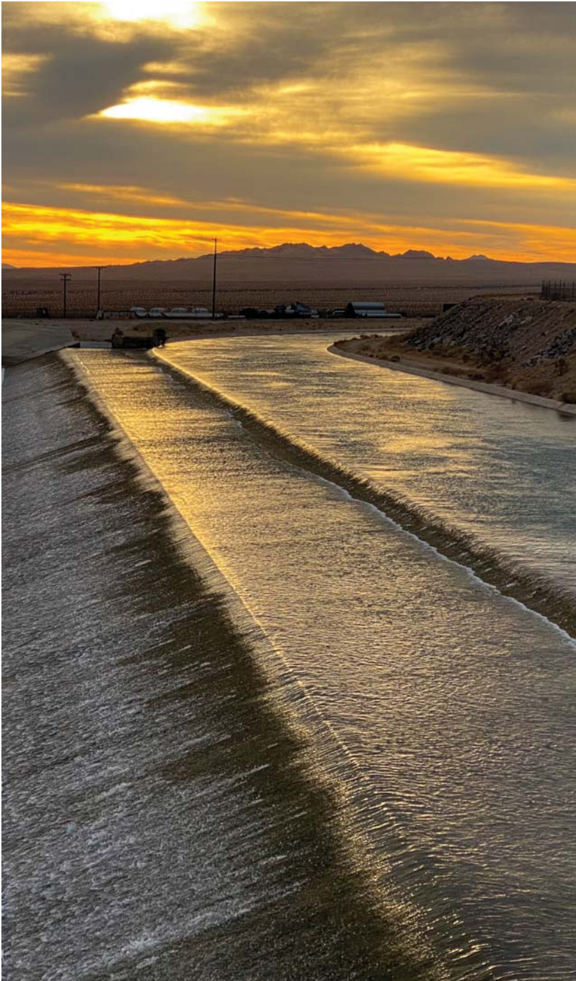
Water from the Colorado River Aqueduct flows over a weir into Iron Mountain Reservoir, before heading to the Iron Mountain pumping plant for delivery to Metropolitan's service area.
