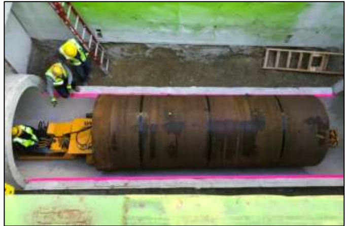
Second Lower Feeder Pipemobile delivering coiled steel liner pipe
