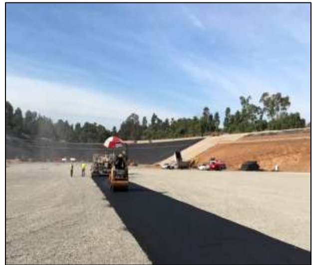
Palos Verdes Reservoir Placement of asphalt paving on reservoir floor
