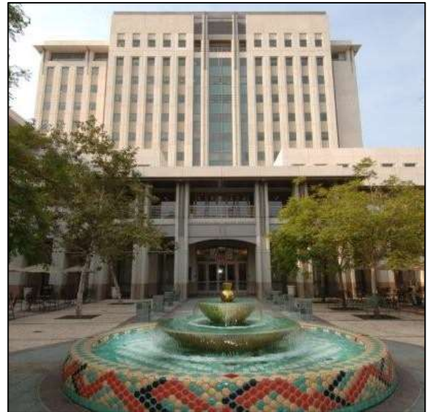
Metropolitan’s Headquarters Building at Union Station
