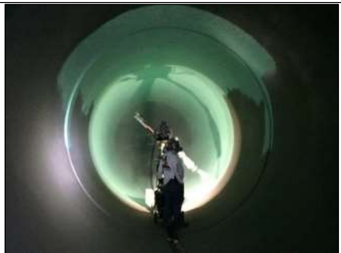
Etiwanda Pipeline Application of polyurethane coating
