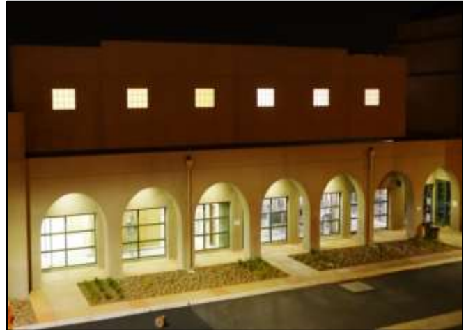
Weymouth Plant Ozone Generation Building
