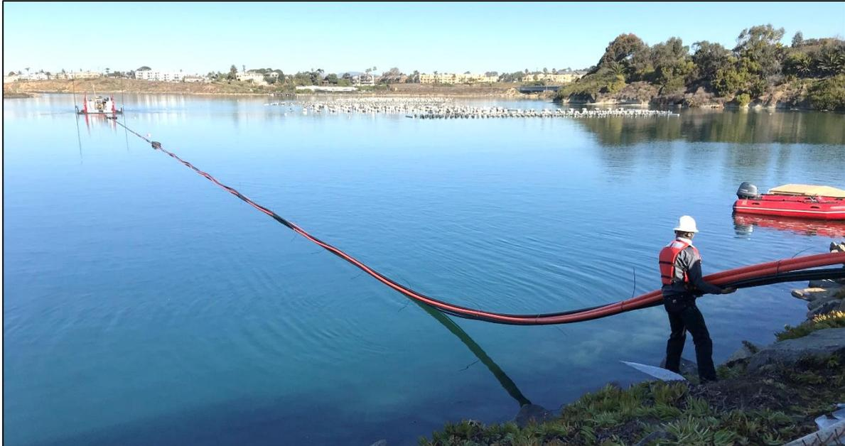
**Figure 8. Installation of the 900-ft long umbilical for the wedgewire screen Pilot Project. Skid can be seen floating offshore in Lagoon while umbilical is paid out; shore end of umbilical was connected to the portable control room after full extent had been paid out.**
