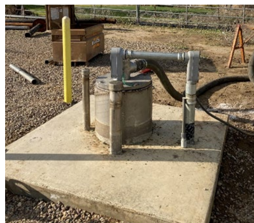
Figure 3-1. Wellhead completed 24-inches above 100-year flood plain.
