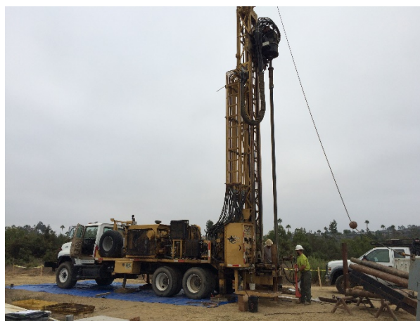
Figure 2-1. Sonic drill rig.
