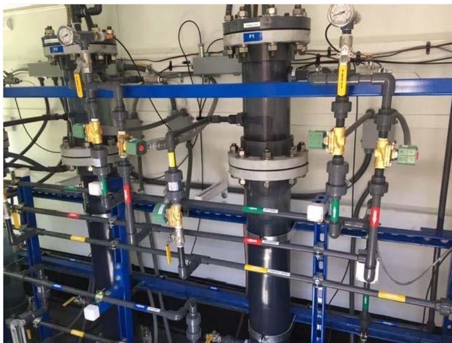
Figure 1: Filter Test Column Setup
