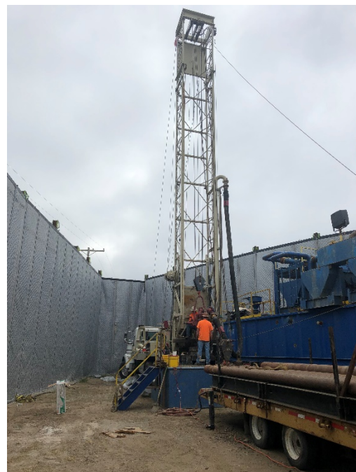
Figure 3-2. Reverse circulation drill rig set up.
