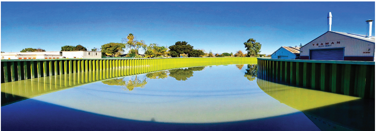
AFTER: SF Creek from East Bayshore.
