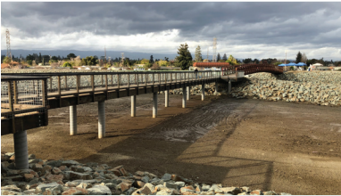
San Francisquito bridge.
