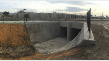
Completed Trestle Bridge along Upper Berryessa Creek.
