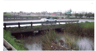
Sunnyvale East Channel (looking south).
