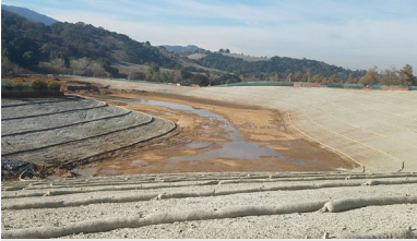
Rancho San Antonio detention basin construction.
