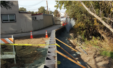
Construction of short-term improvements at the Rock Springs neighborhood.
