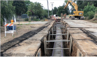
Main Ave. pipeline installation.
