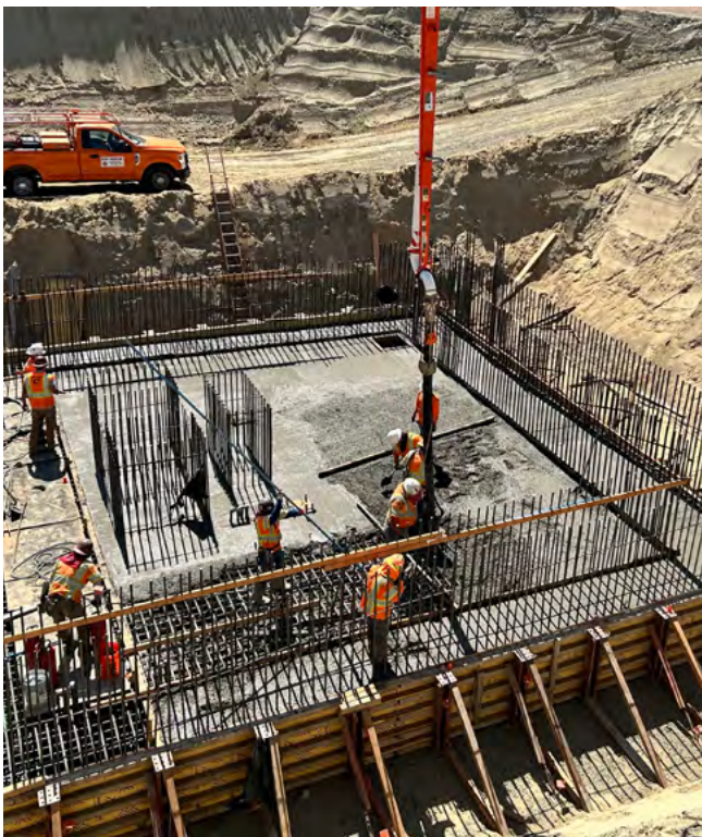
Valve vault foundation for Badlands Tunnel Project
