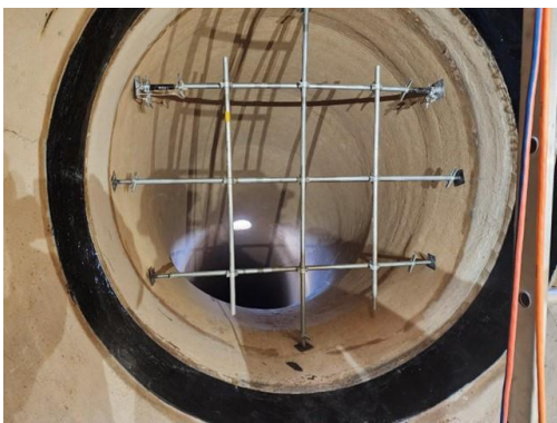
Completed Delivery Line 2 transition Joint
