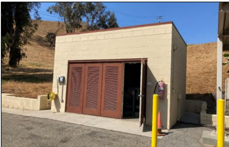
Standby Generator Building, Facing Southwest.
