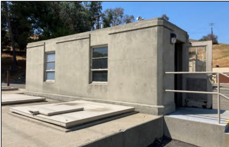
Junction Structure Access and Roof, Facing South.
