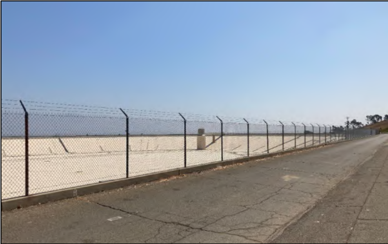
Reservoir and Access Road, Facing Northeast.
