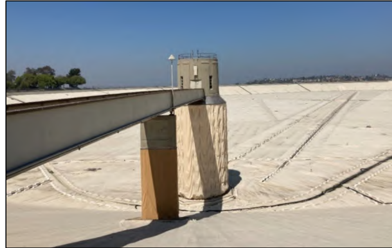
Reservoir Cover, I/O Tower and Access Bridge, Facing West.
