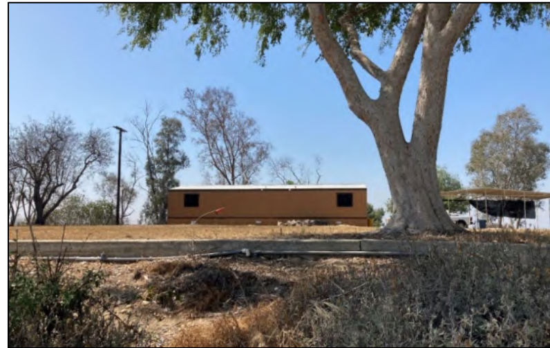
Construction Trailer Office, Facing South
