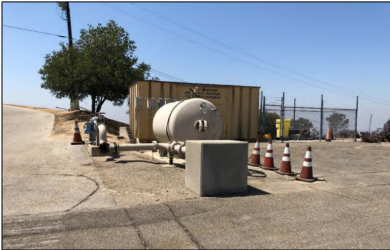
Surge Tank, Facing South
