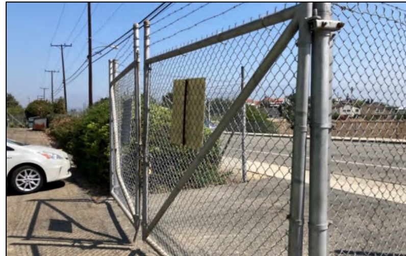
Access Gate and Chain Link Fencing, Facing Northeast
