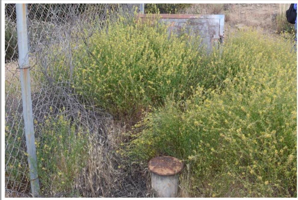
WWF1 Station 1415+37 and 1415+42, exposed valve, facing north/west.
