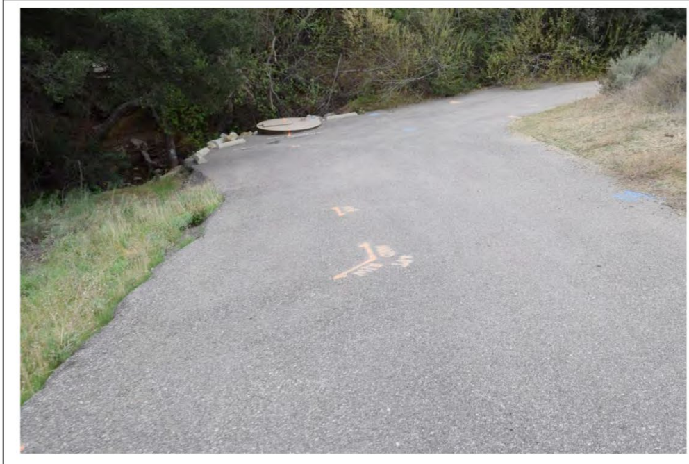
WWF1 Station 1407+45, facing south/west.
