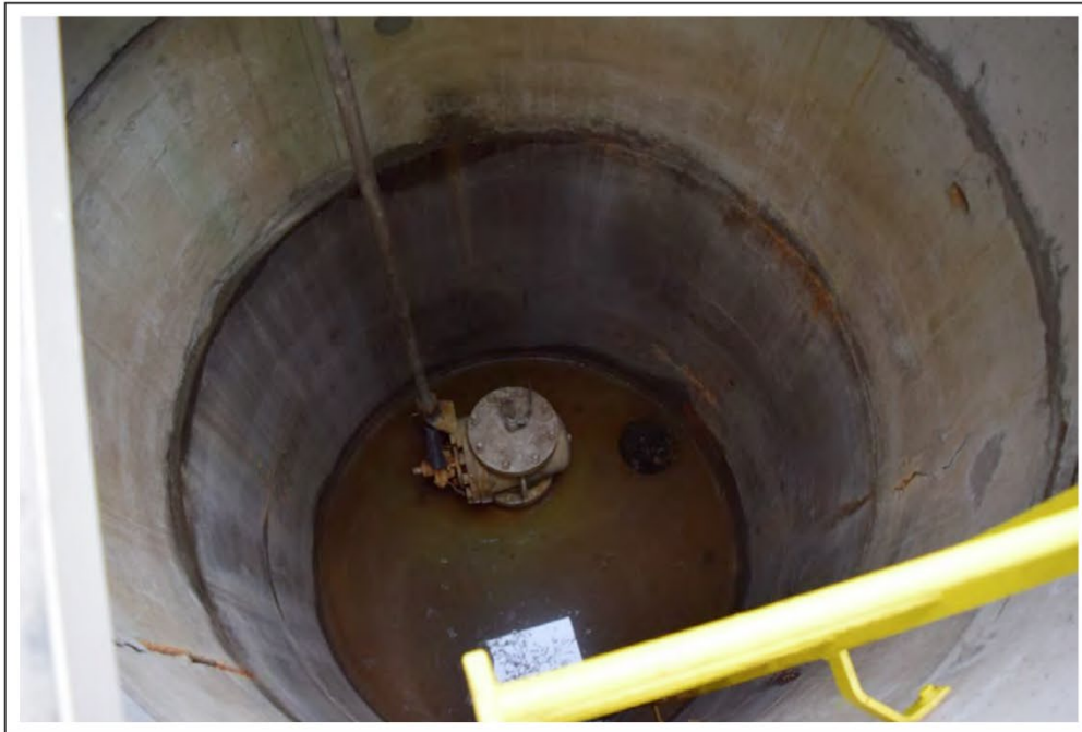
WWF1 Station 1407+45, manhole interior.
