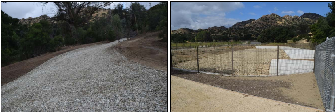
Figure 5 - Stone Lined Stream and Park Detention Basin
