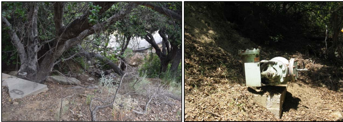
Figure 2 - WVF1 STA 1407+45 at Stream Crossing and WVF1 STA 1416+33 at Stream Bottom
